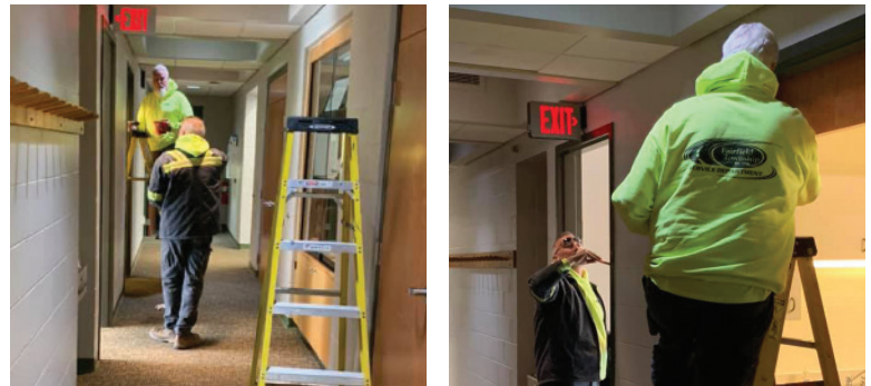
Administration building remodeling
